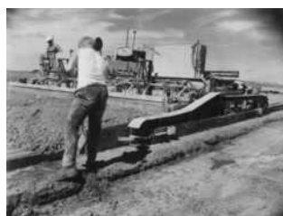
Minnesota Historical Society Construction being done on I-94.
