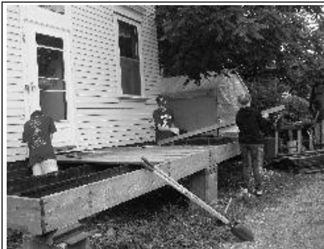
An Urban CROSS team, working on a neighbor's deck.
