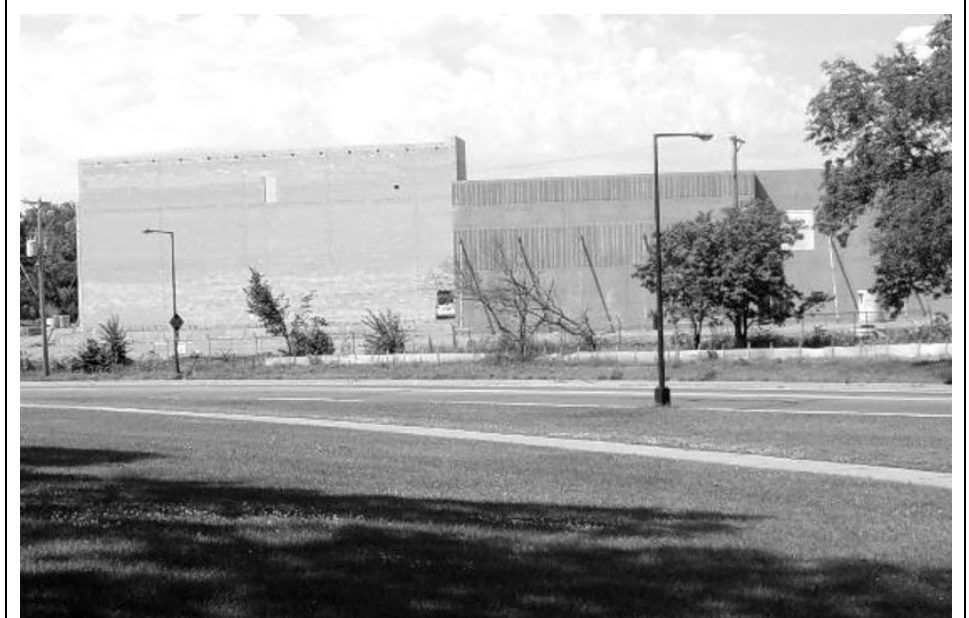
Baldinger Bakery going up on the north end of Johnson Parkway
