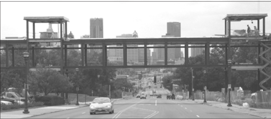
Looking down 7th St. towards downtown as the skyway to the new Metropolitan State/Community library was being constructed last year.
